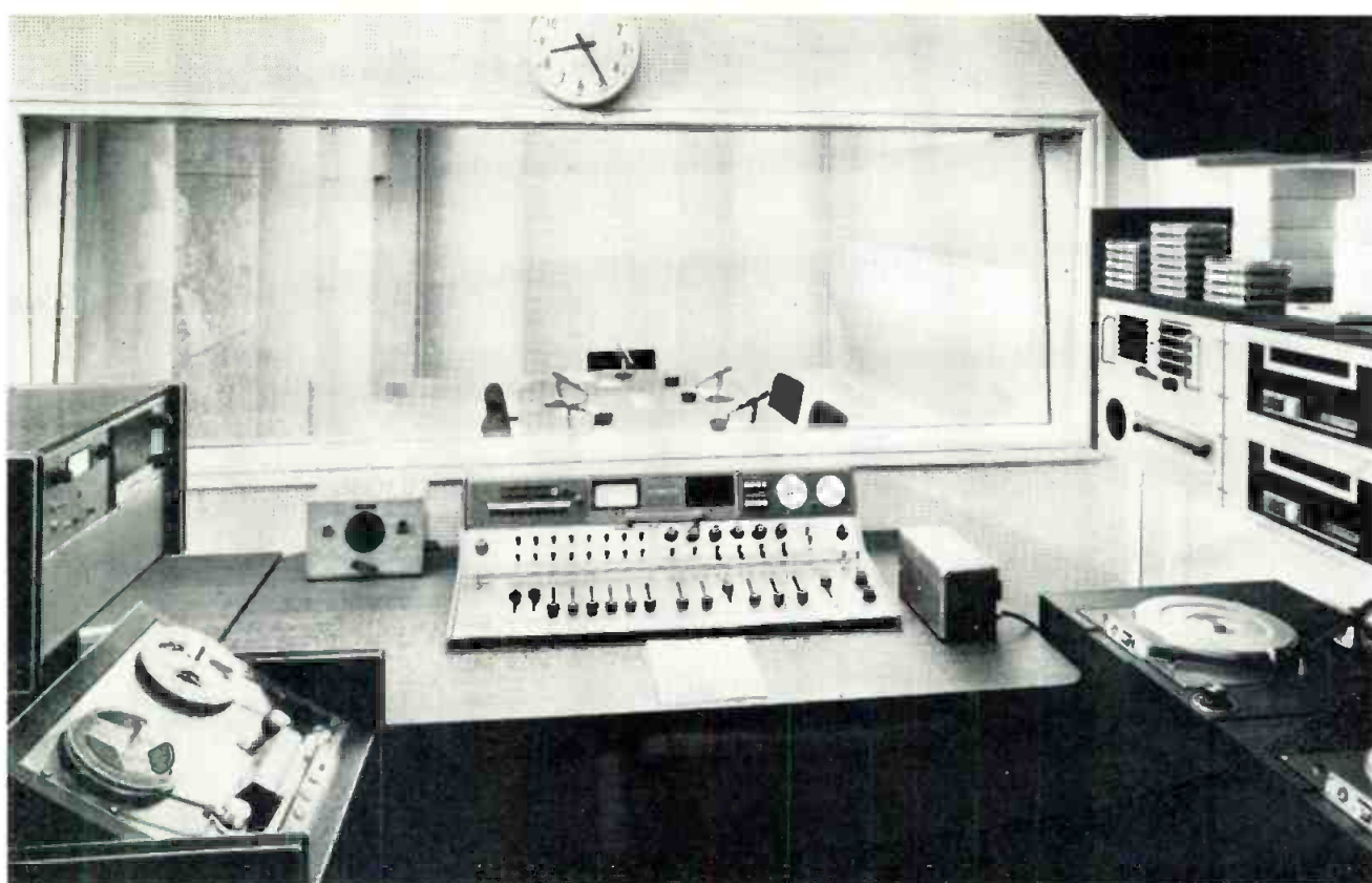
This radio control room has a state-of-the-art console with 15 slide-wire pots, inbuilt clock, and dial-remote system.
